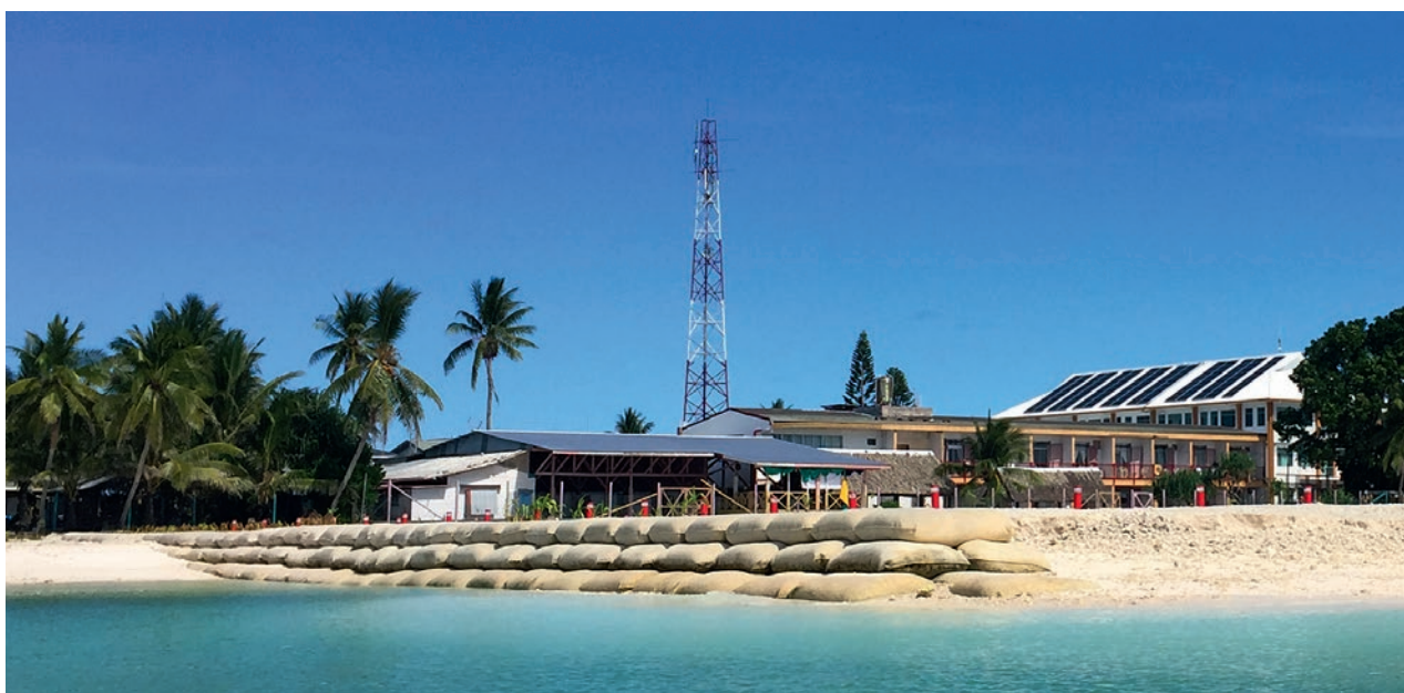
Measures to adapt to climate-related sea level rise by building artificial sea walls in Tuvalu, South Pacific
