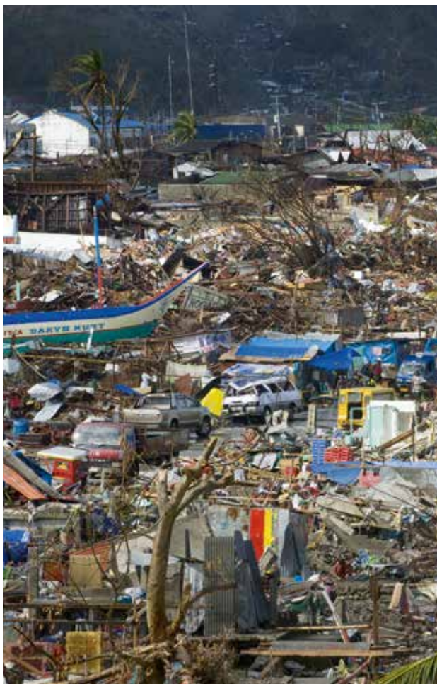
Tacloban City in the Philippines was heavily devastated by Typhoon Haiyan, which made landfall in the country in November 2013.
