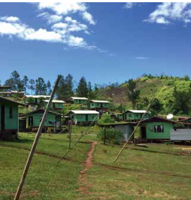
Vunidogoloa village in Fiji has been relocated to higher ground due to sea level rise. The old site is regularly flooded and does not provide a safe home for the 156 villagers.
